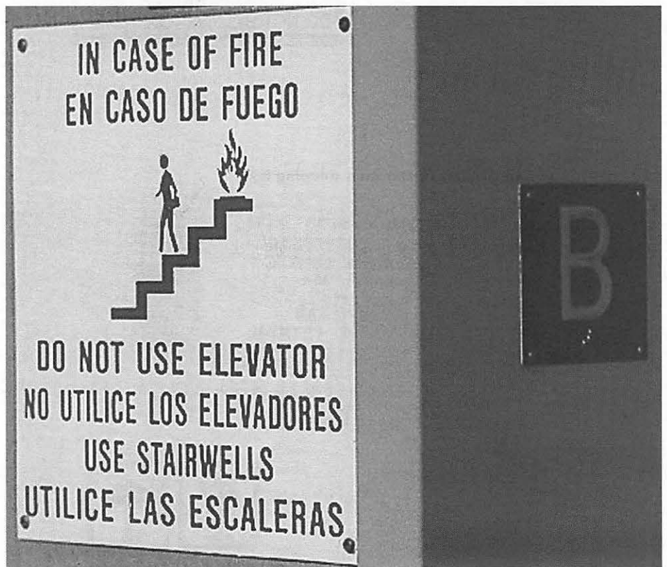
1-21: Poorly placed fire safety sign
