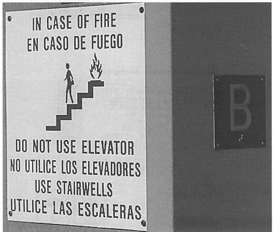
1-21: Poorly placed fire safety sign
