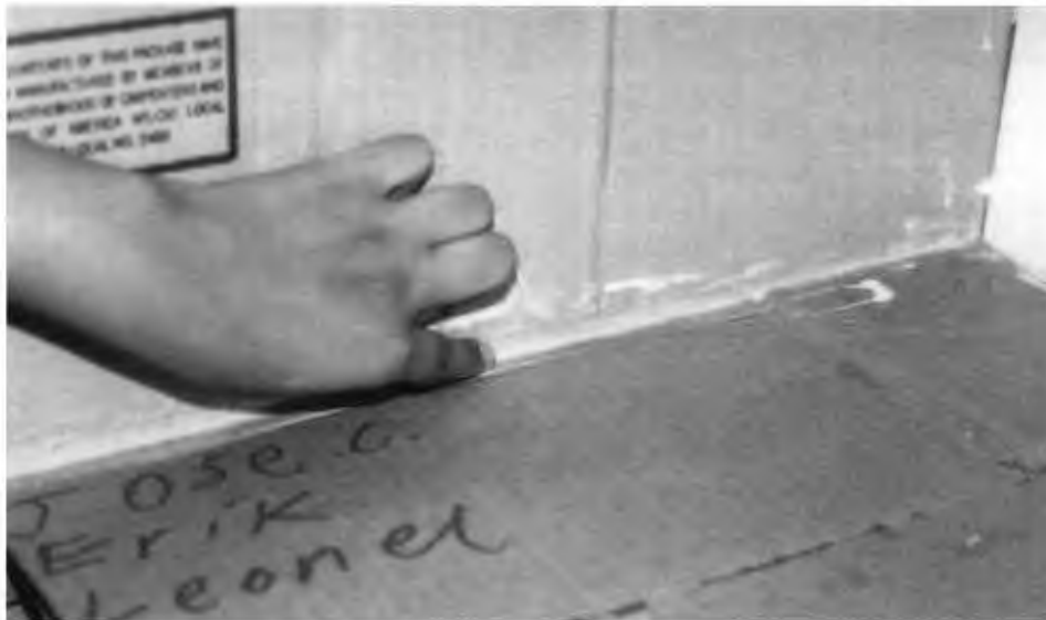
4-44: Gluing shelf to support strip
